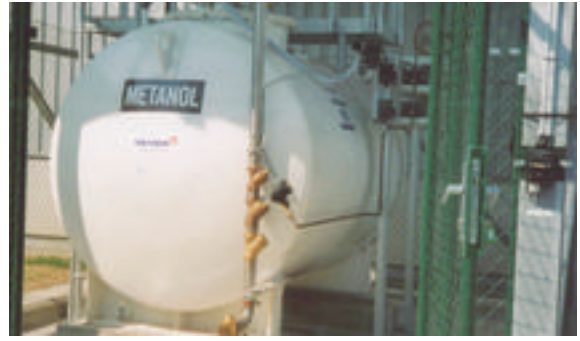
Methanol is stored outdoors.
