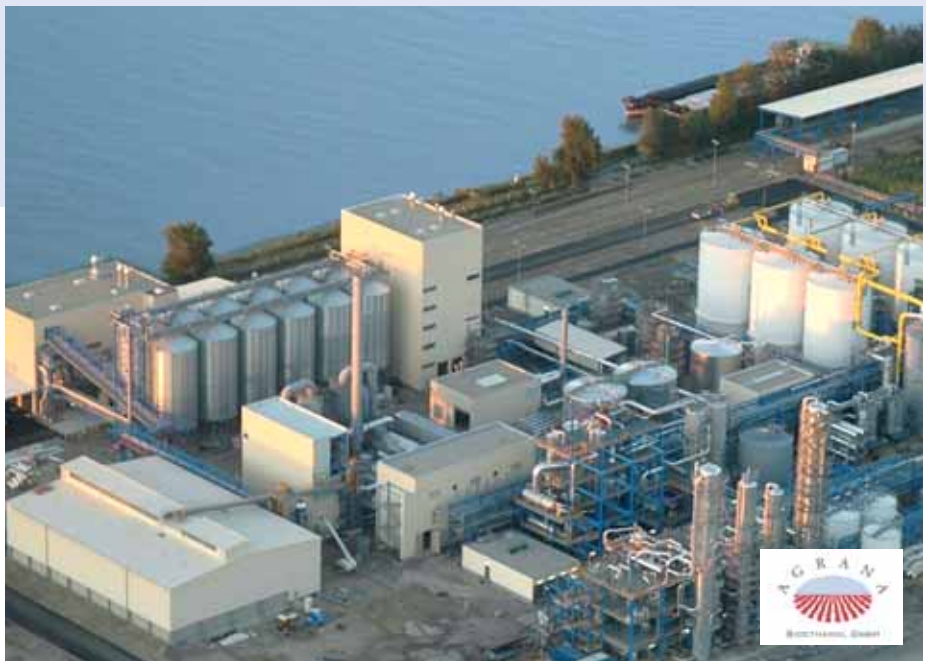
In one of the largest European bioethanol production plants in Pischelsdorf, Austria, nitrogen from Messer protects against explosions.
