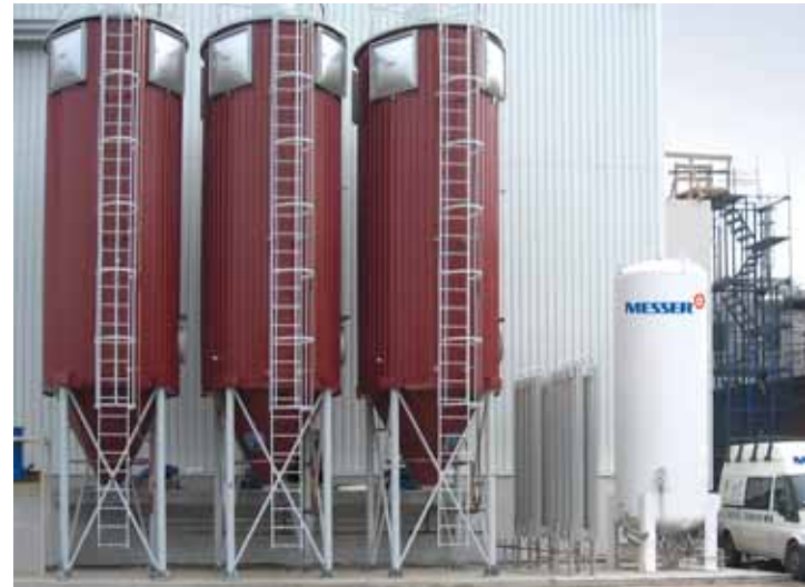
In Lublin, Poland, dried sewage sludge is stored safely in silos.
